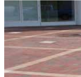
Concrete with precast concrete bands
