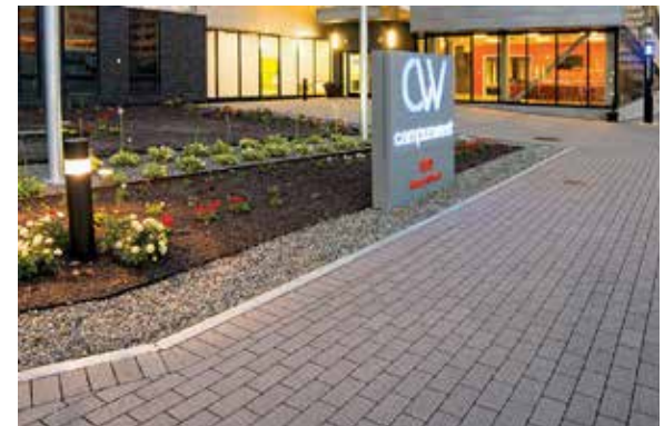
Permeable precast concrete pavers
